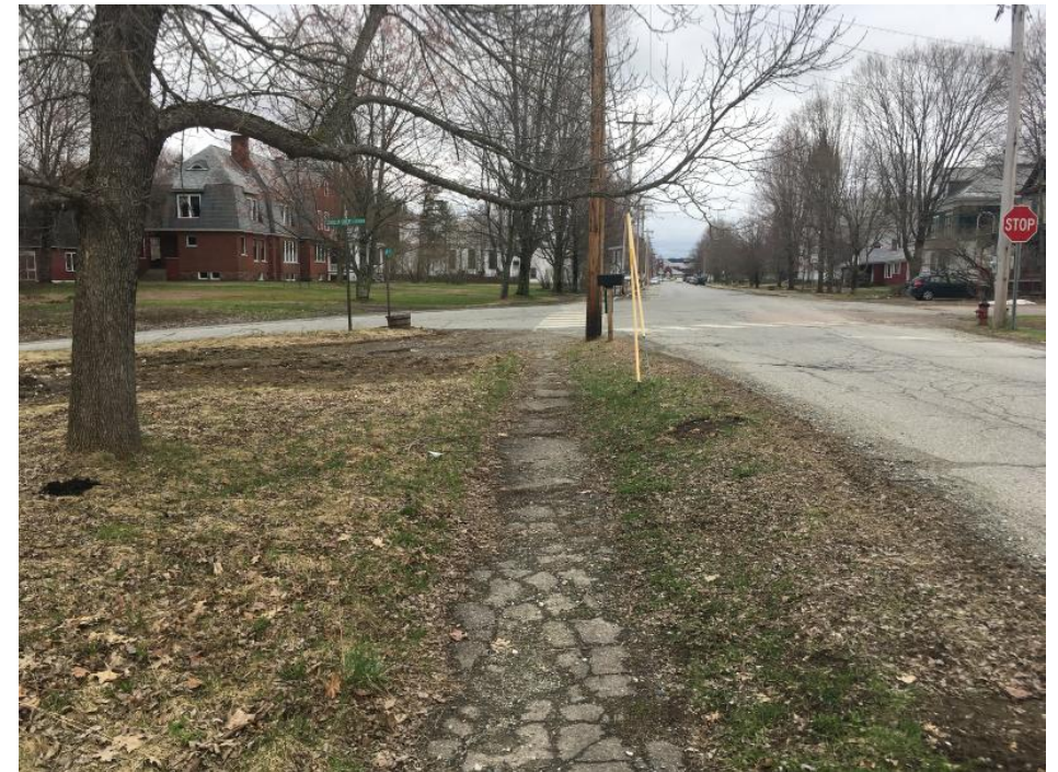
4 foot asphalt sidewalk on West Main Street
