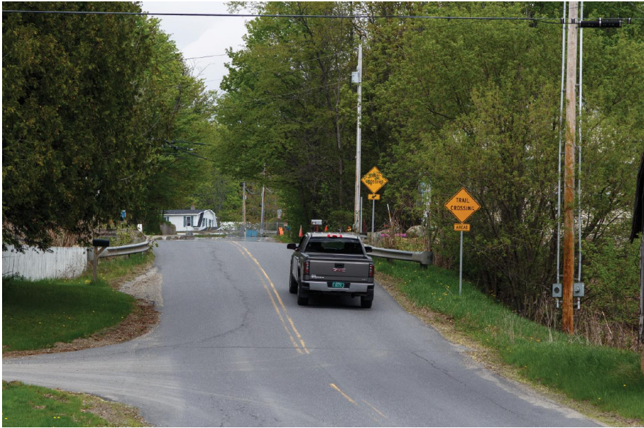
Looking at the Depot Street LVRT Crossing from the south
