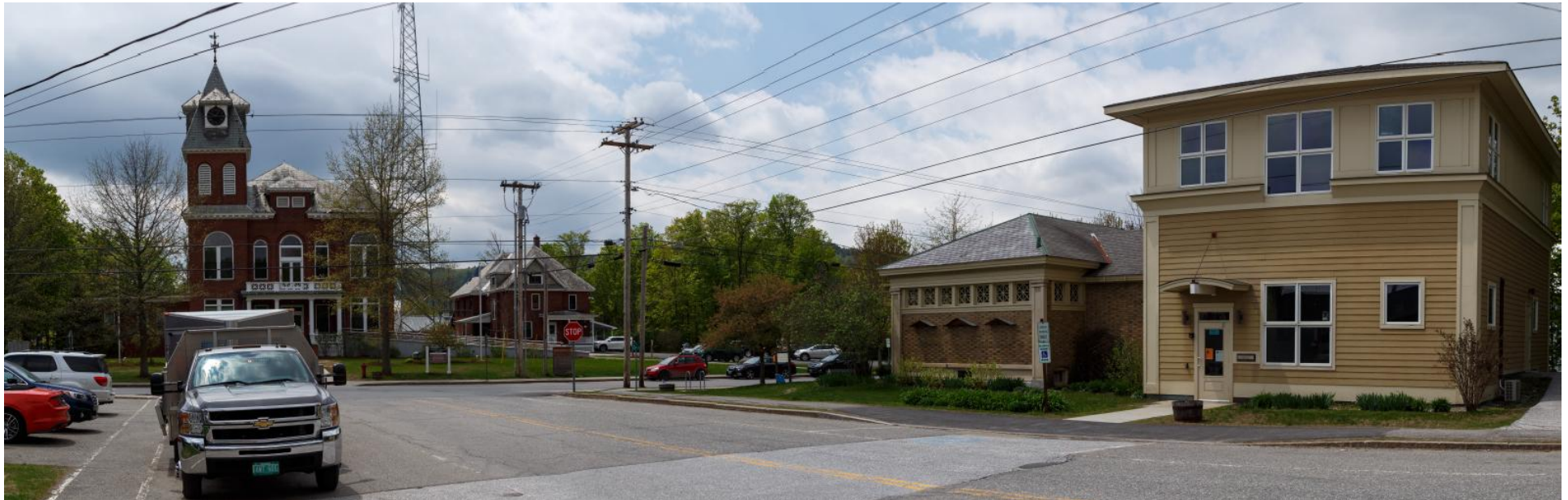
Painted pedestrian lane (left) and asphalt sidewalk (right) on Church Street
