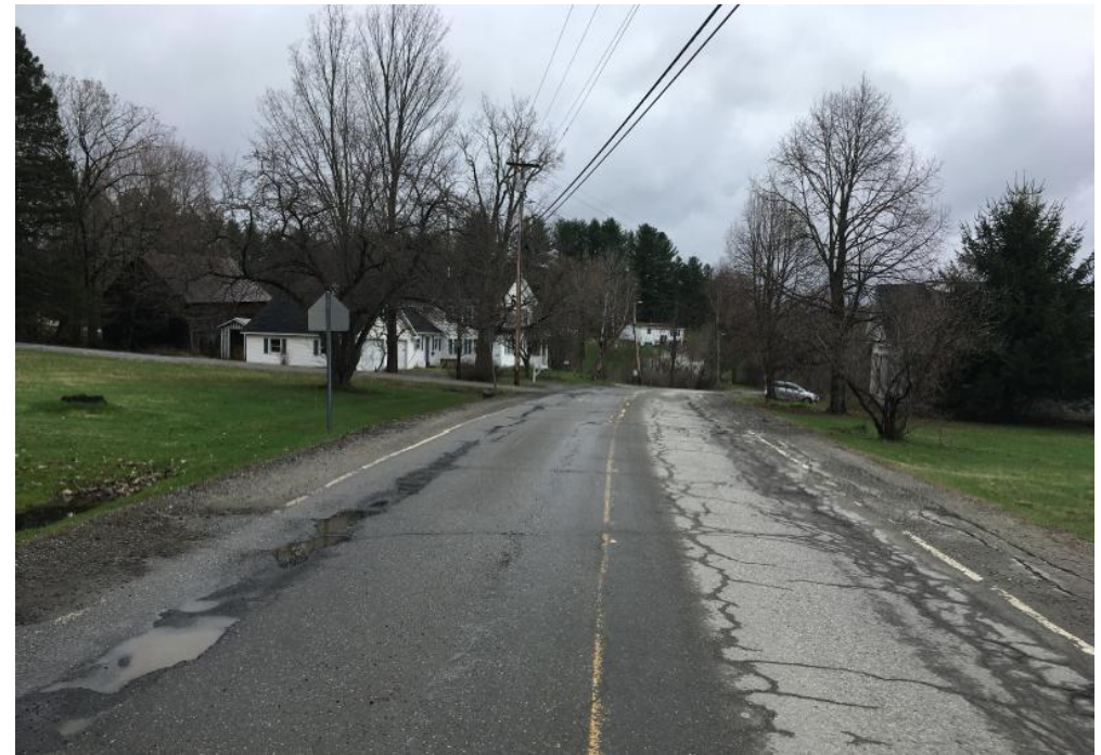
Looking east on E Main St near designated village boundary
