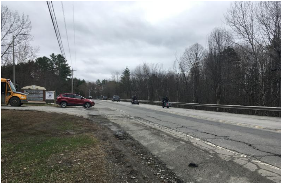
Looking east at the VT15 and LUHS intersection
