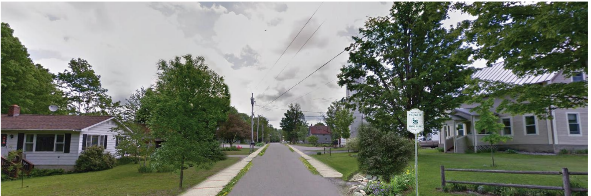
Looking east on West Main Street - with sidewalks, a rain garden, and a gateway sign
