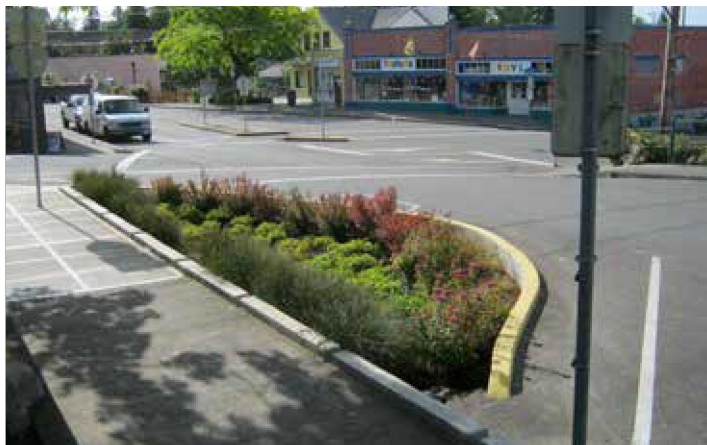
Figure 25 (above). Stormwater curb extensions cross section from Great Streets BTV
