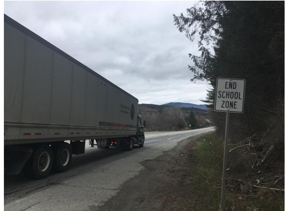
Looking west on Route 15 towards Black Farm Road
